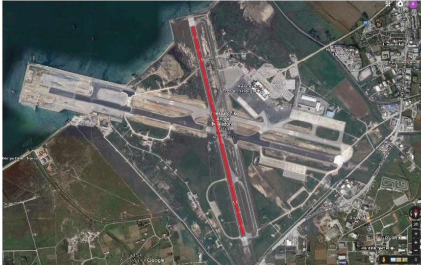
Figure 4: The runway of the airport of Thessaloniki used for coast-down testing
