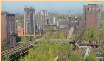
Nature taking over industrial relics (abandoned coal processing plant: Kokerei Hansa, Dortmund, Germany). Photo: Ingo Kowarik
